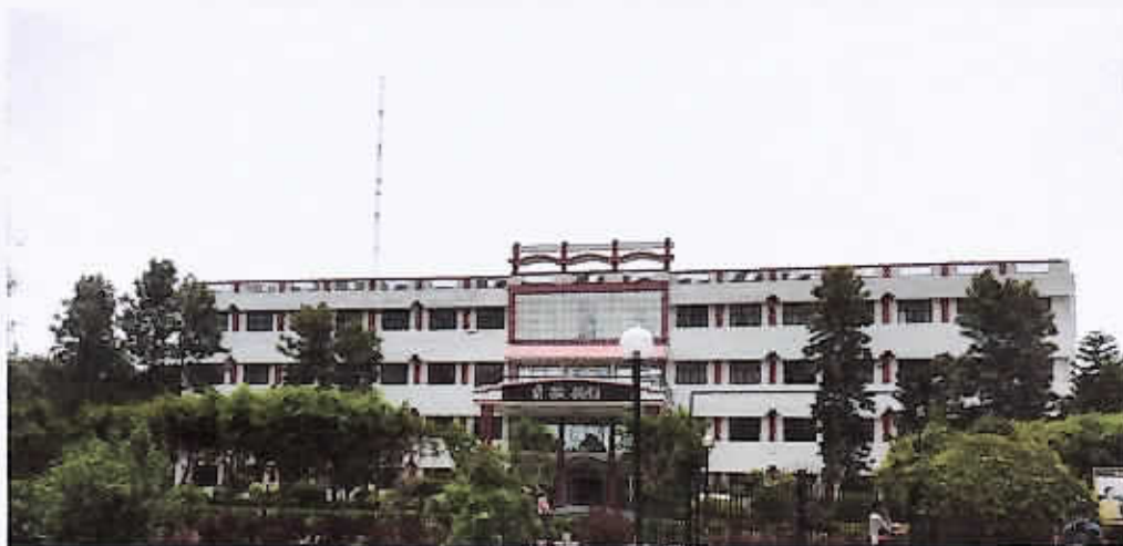
CAMPUS (MAIN GATE BLOCK 'B')
